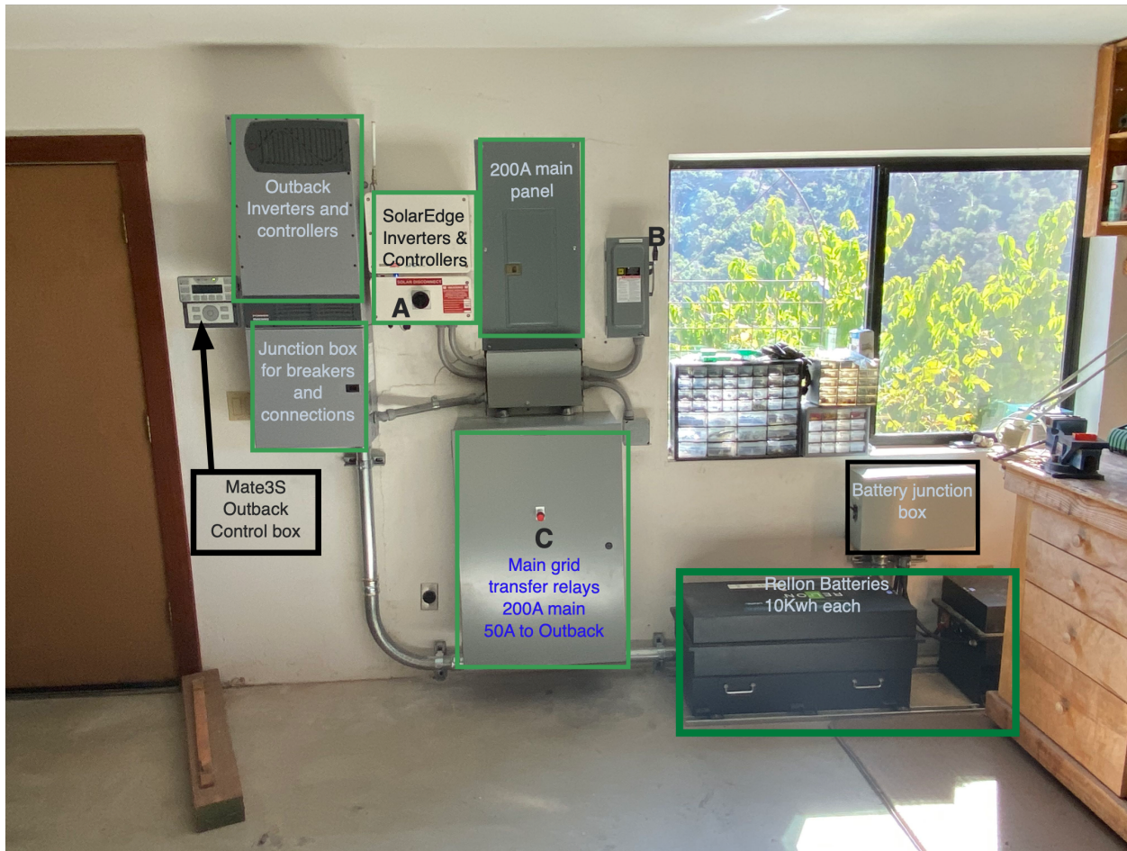
Figure 1. Components of the backup system, installed by Sun Pacific Solar Electric.
